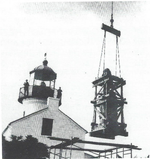
A crane from the Hazard Company moved the de Bree statue to the new Visitor Center in 1966. Author's collection.
